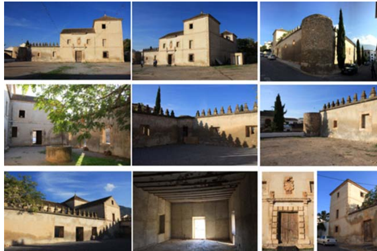
Figure 2. House Palace of Padul's Earl. Current status
